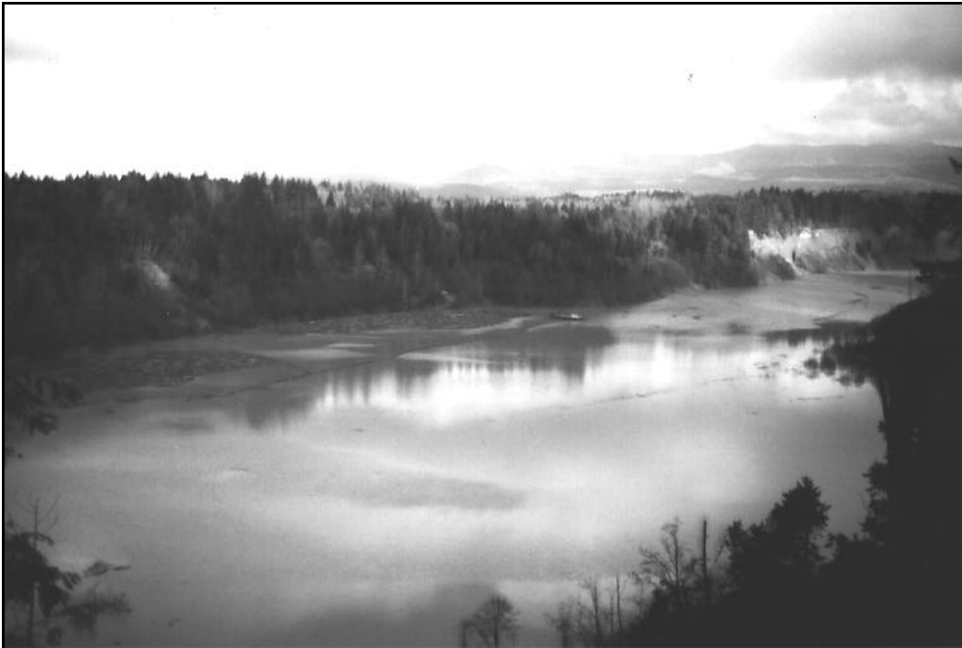
Photograph 2.4 Lower Debris Basin with Pool
