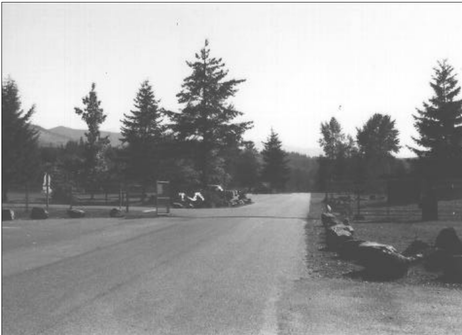
Photograph 6.1 Project Entry Road
