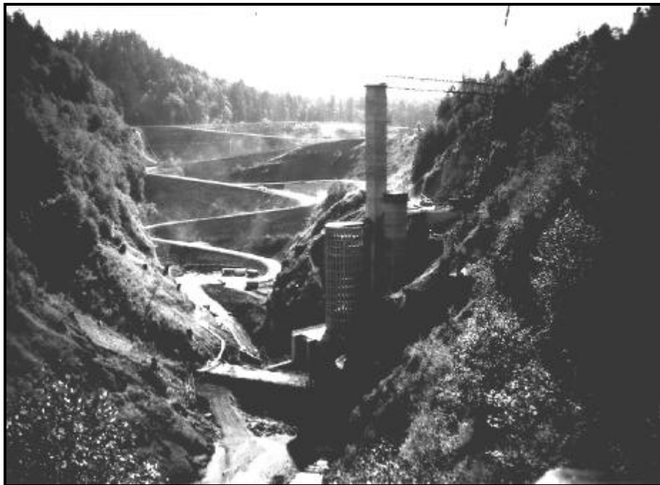
Photograph 2.1 Upstream face of Mud Mountain Dam
